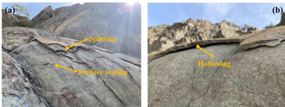
Figure 2 Typical Diseases in Helankou Rock Art: (a) Splitting with Parts of the Surface already Detached; (b) Hollowing with the Surface Separating from the Rock Body.
